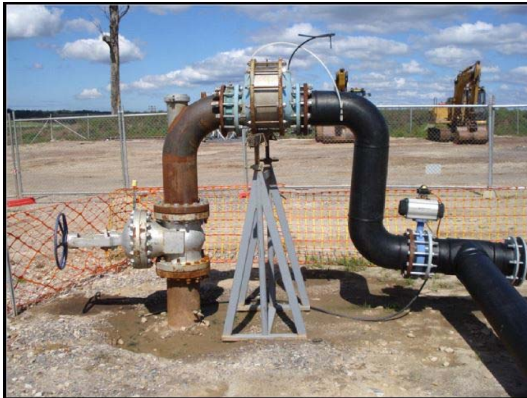
Figure 24 : Typical Connection to Vertical Drainage Wells (Cardno, 2011)
